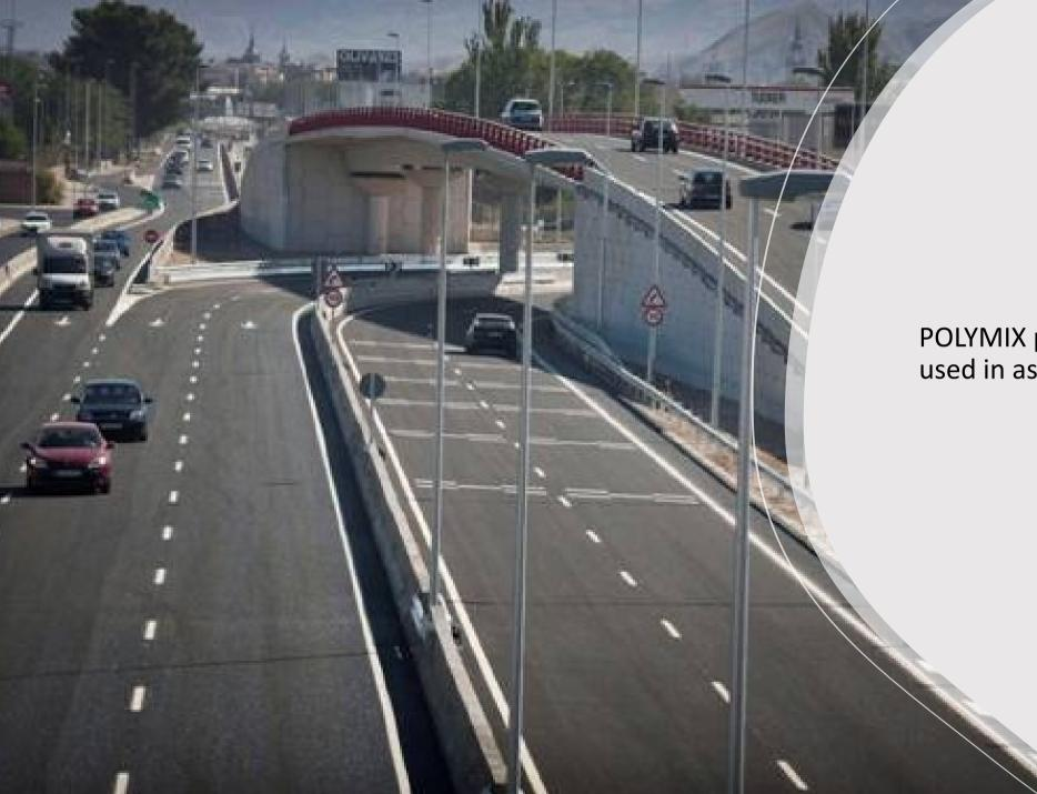
POLYMIX project: plastic waste used in asphalt
